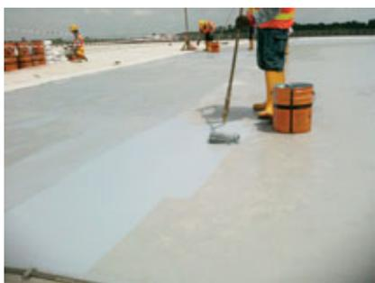
Fig. 12.1 – Application of liquid-applied membrane using roller.
