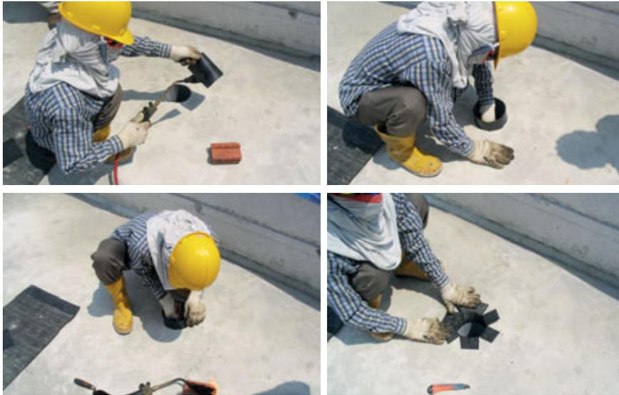
Fig. 12.8 – Wrapping around pipe penetration.
