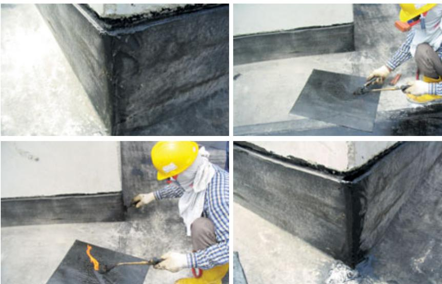
Fig. 12.7 – Overlapping and sealing at corner.
