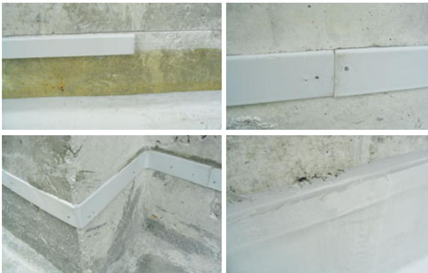
Fig. 12.10 – PVC coated strips for perimeter terminations.
